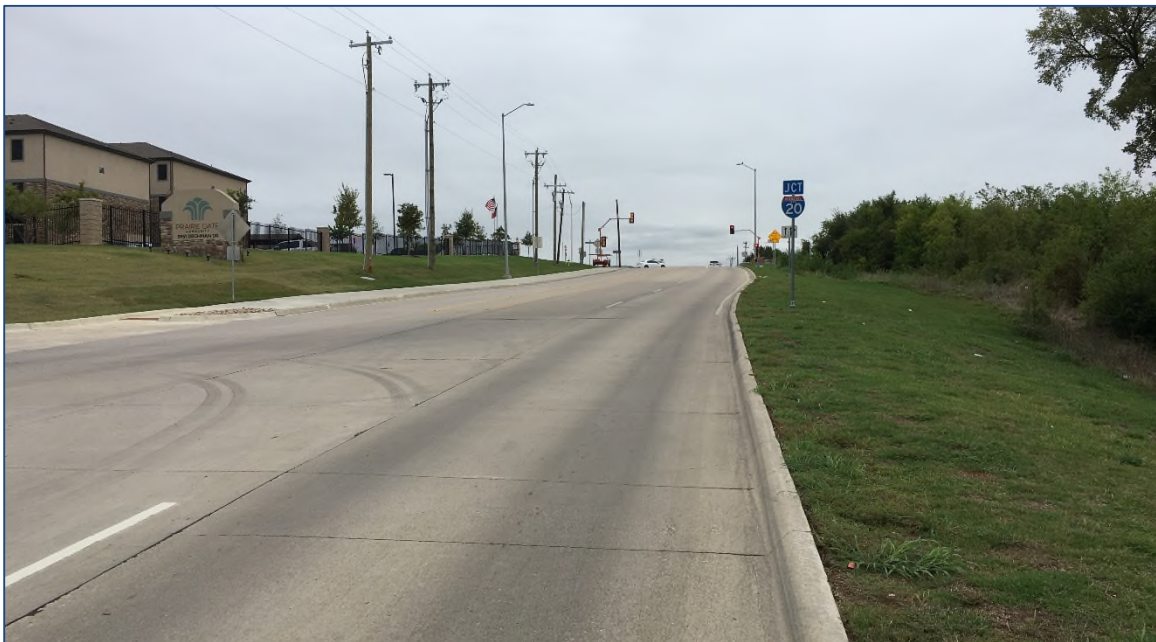
Dechman Drive & Project Access - looking south
