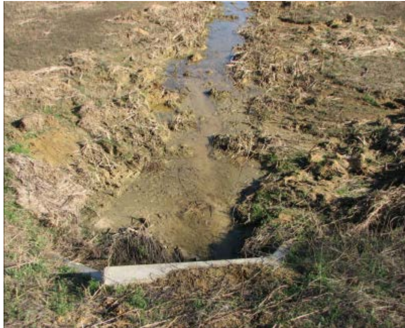
Picture XI-2 – Example of RipRap/Scour Criteria (Photo ID 1613)
