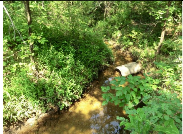
Looking upstream from 1153 there was a second segment of concrete pipe.
