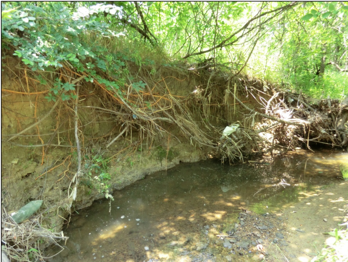
Figure 4.7 Looking downstream at severe bend scour near cross section 3177
