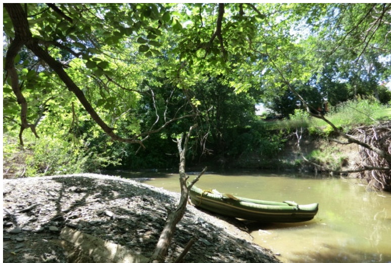
Figure IX-12: Bank Erosion at Cross Section 9-4
