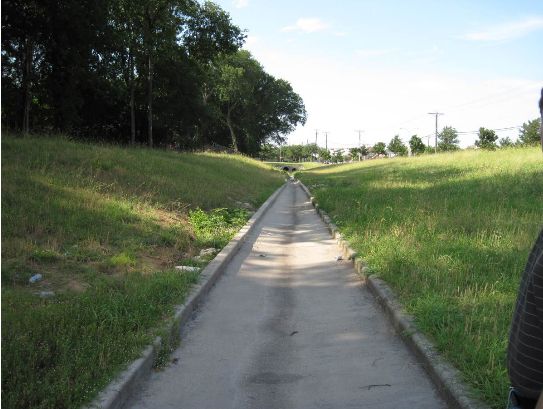
Figure X-24: FC Detention Pond No. 21: NE Corner of Robinson and Bardin Roads
