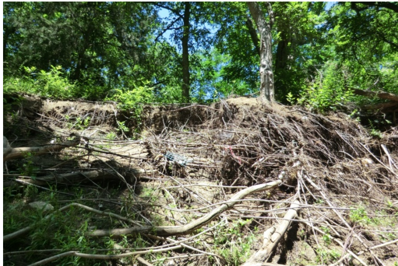
Figure IX-8: Bank Erosion at Cross Section 200+46
