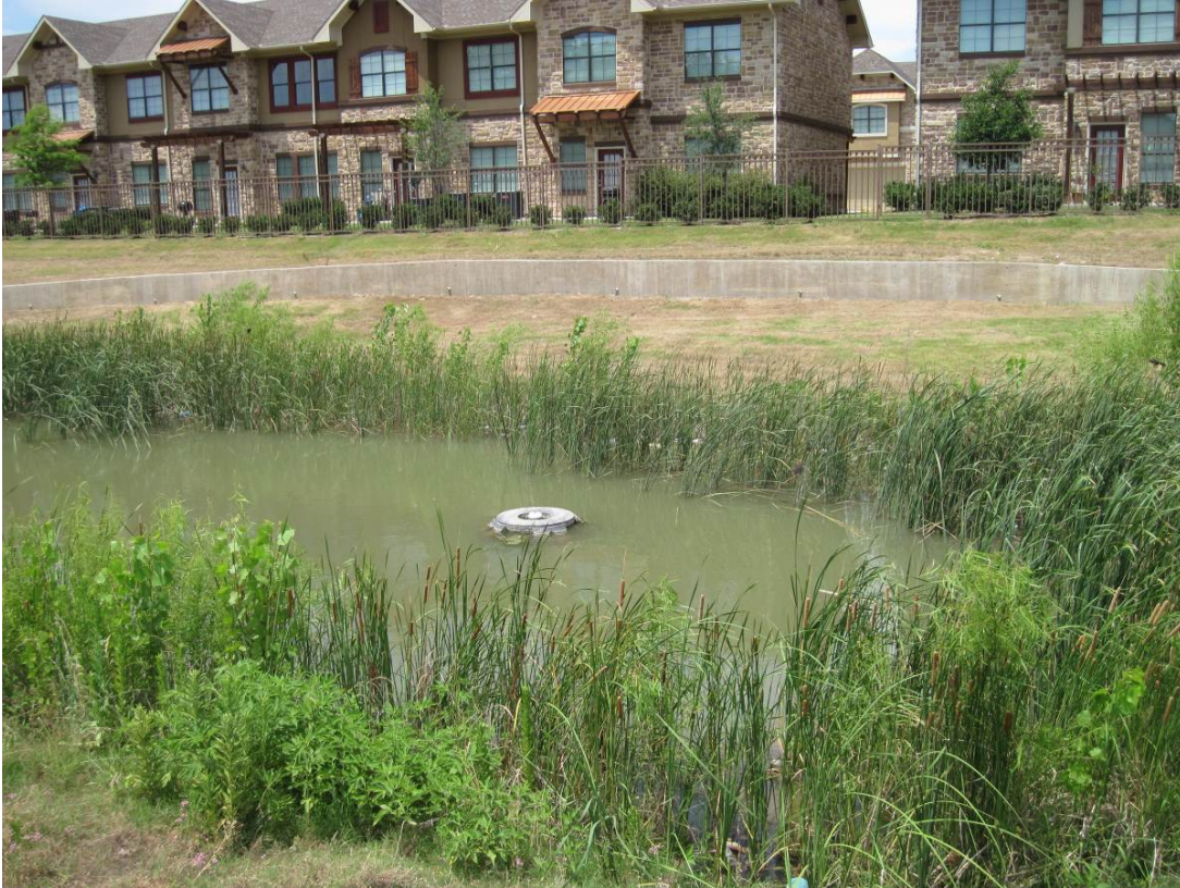
Figure X-14: FC Detention Pond No. 12: Apartments off Magna Carta Boulevard
