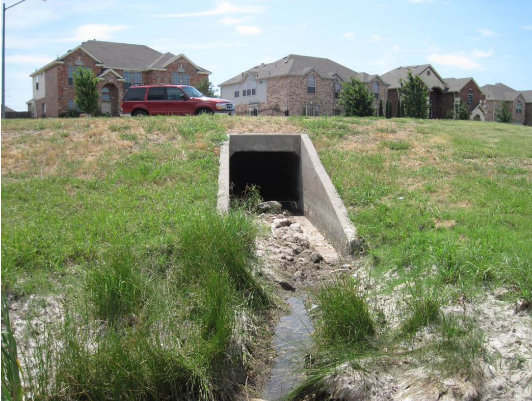
Figure X-20: FC Detention Pond No. 17: Between Conrad Lane & Brewster Court
