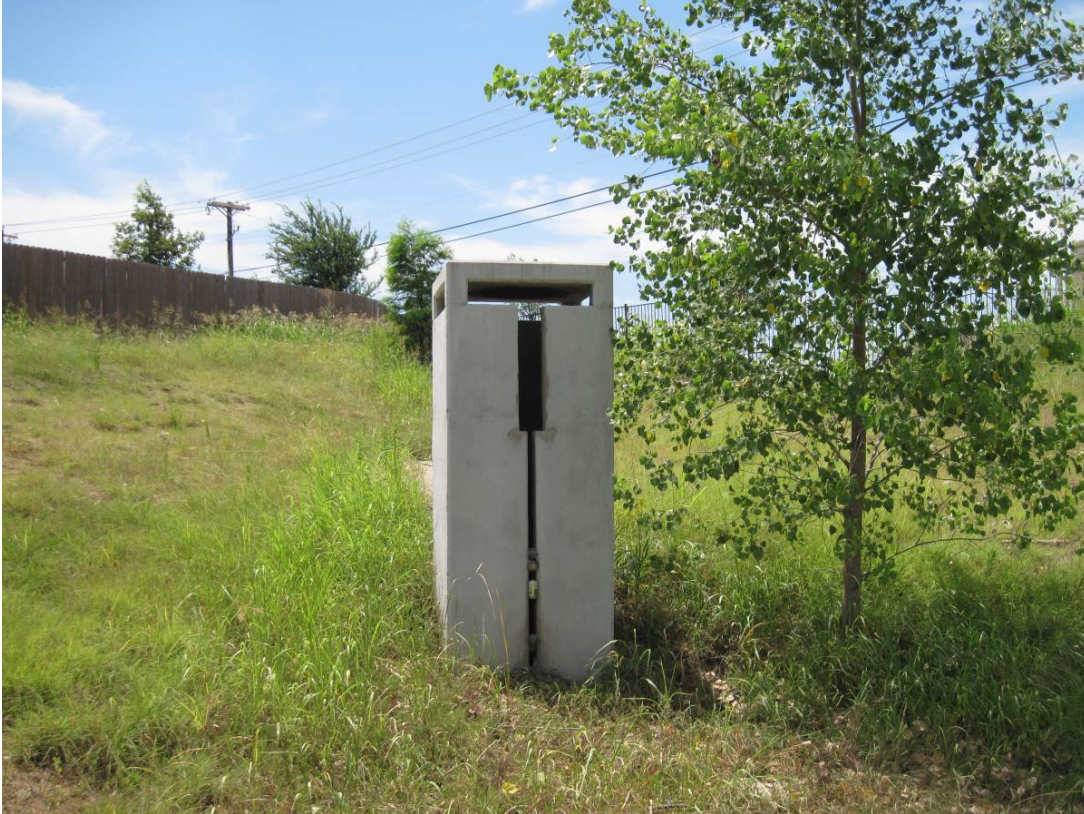
Figure X-16: FC Detention Pond No. 14: Eastside of Magna Carta just north of W Camp Wisdom
