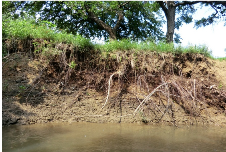
Figure IX-6: Bank Erosion at Cross Section 321+67
