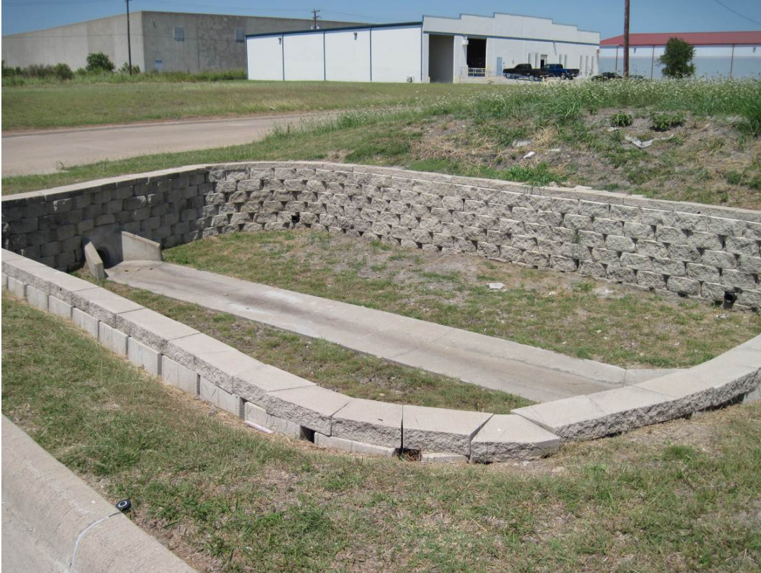
Figure X-12: FC Detention Pond No. 10: Off Eagle Drive
