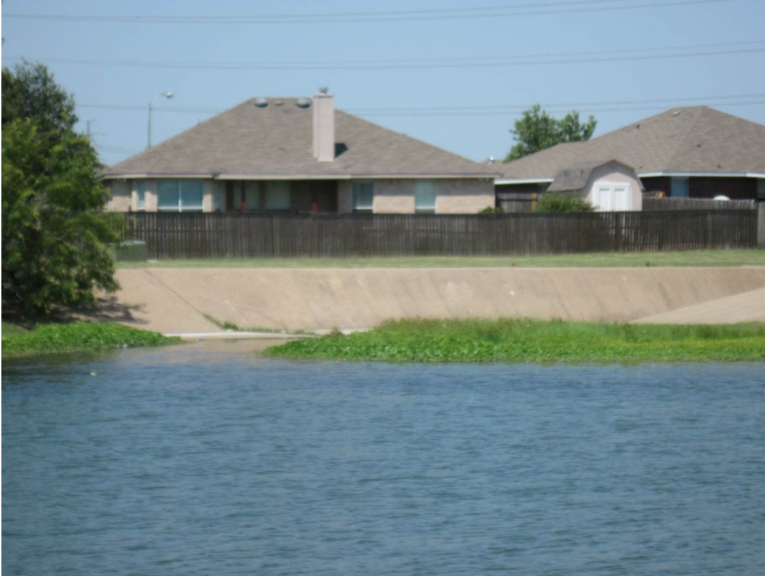
Figure X-8: FC Detention Pond No. 7: Small Pond Behind Southwood Trail
