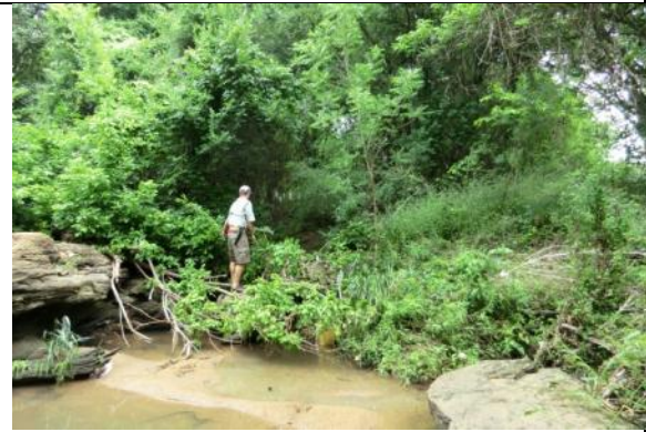
At 38331 outfall, gully erosion
