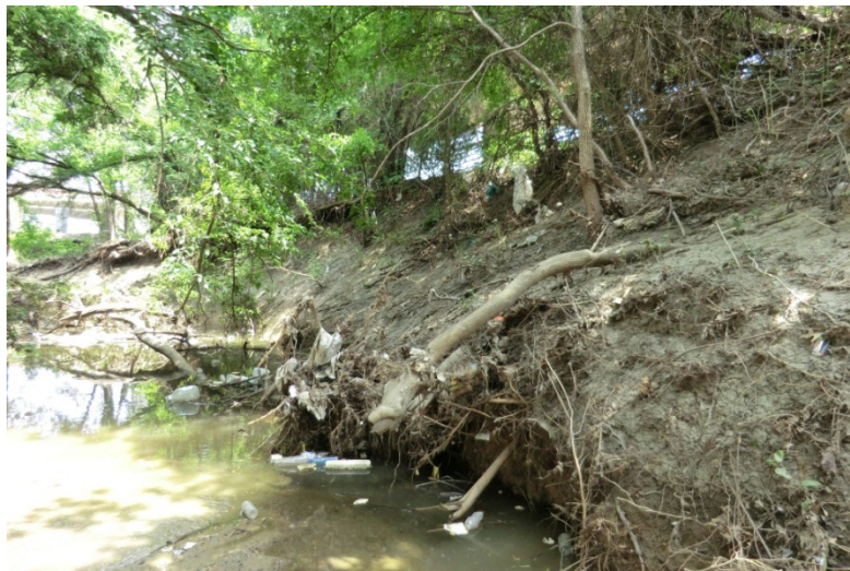
Figure IX-15: Bank Erosion at Cross Section 24+63
