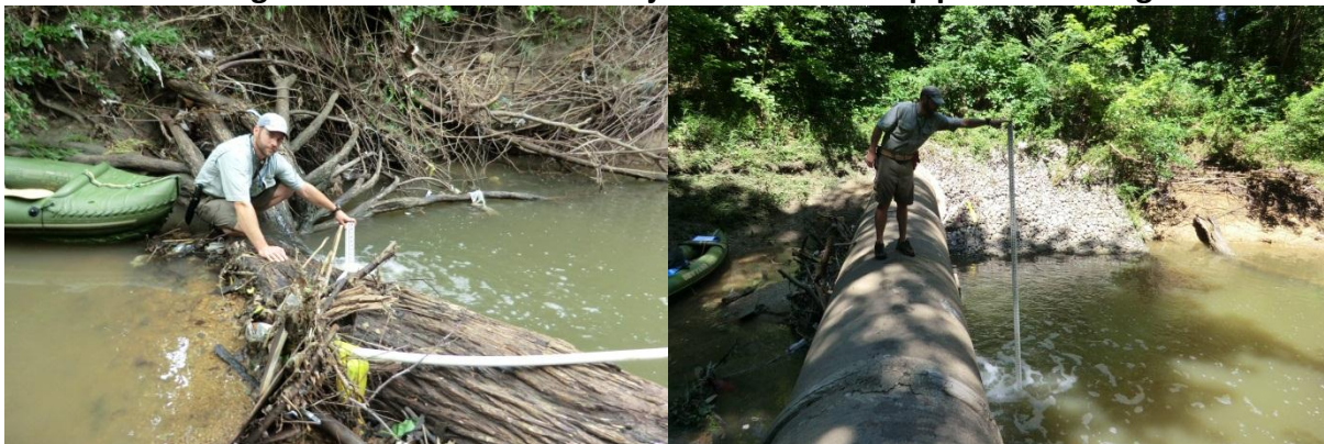
Figure 3.5 Photos of LWD jam and an aerial pipeline crossing
