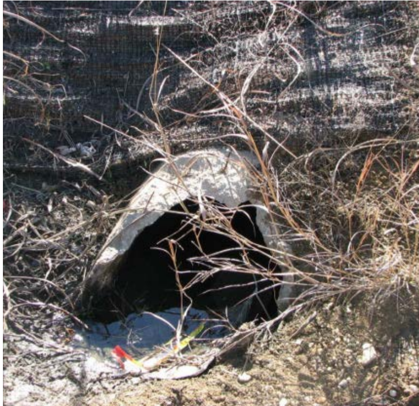
Picture XI-4 – Example of No Headwall Criteria
