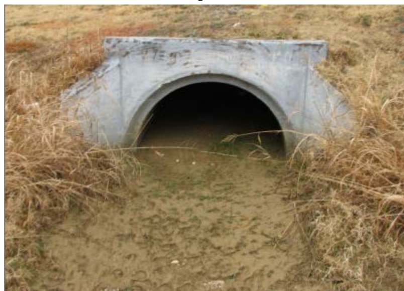
Picture XI-3 – Example of Siltation Criteria
