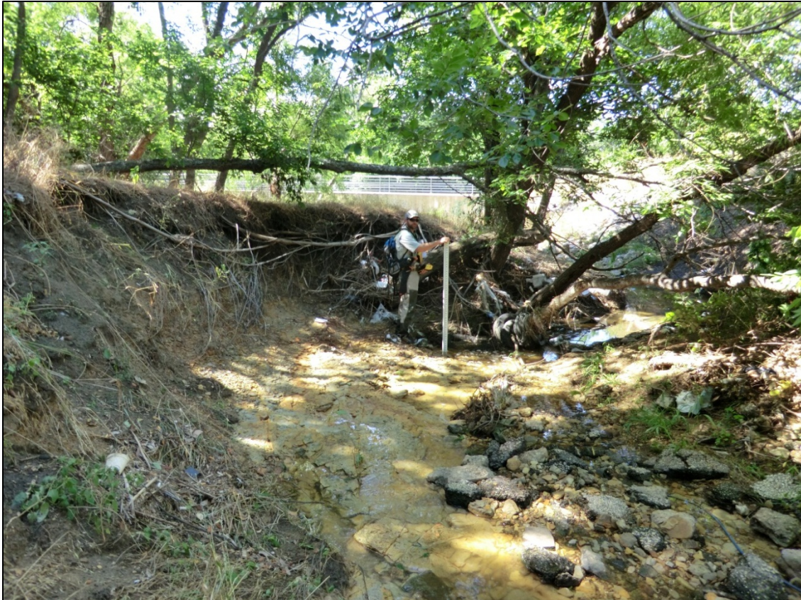
Figure 4.5 Looking downstream at bank erosion on the left bank near cross section 4526
