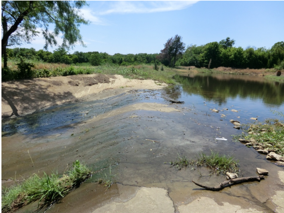
Figure X-2 – On-Channel Pond: Spillway Upstream
