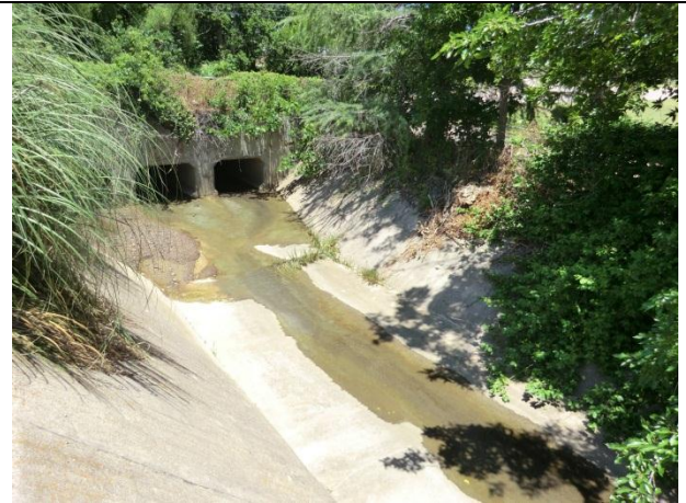
Upstream view from 2151 shows a concrete channel.
