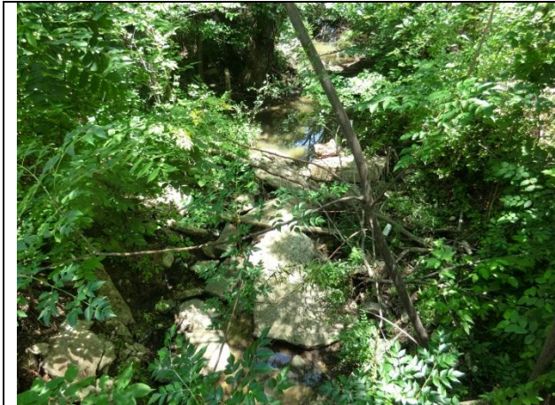
Downstream from 2809 there was concrete rubble in the channel below a pedestrian bridge.
