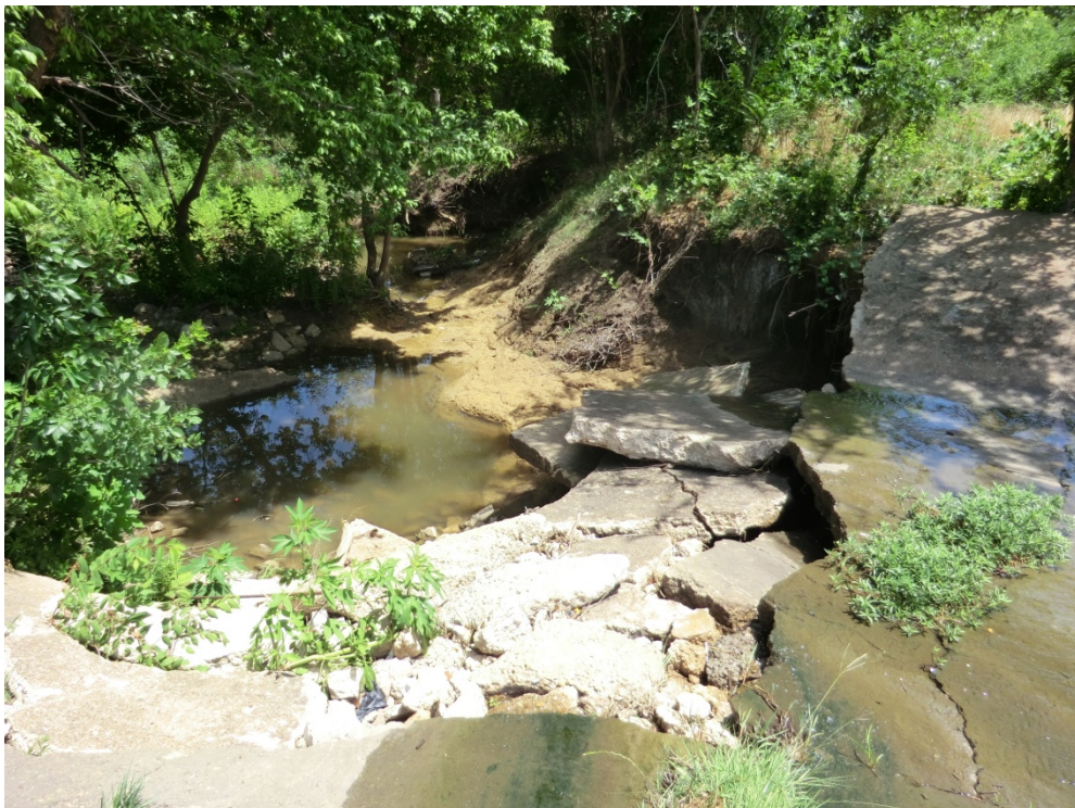
Figure X-3 – On-Channel Pond: Spillway Downstream
