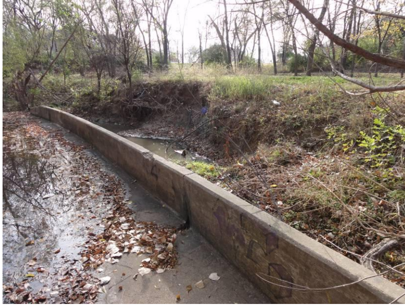
Figure 29. Channel jumps concrete liner and is scouring bank.
