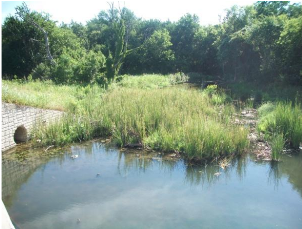
Carrier Pkwy Crossing: Looking Downstream
