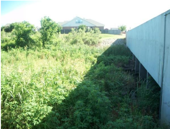
Bardin Rd Crossing: Downstream Face
