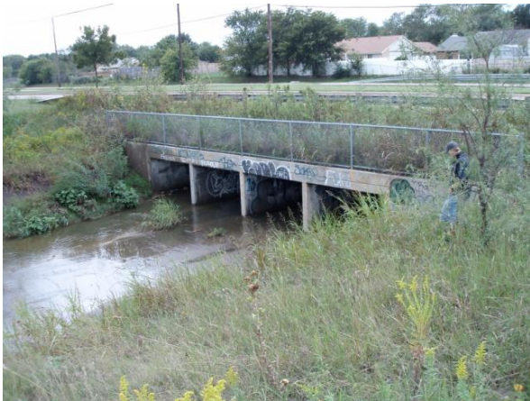
Robinson Rd Crossing: Downstream Face
