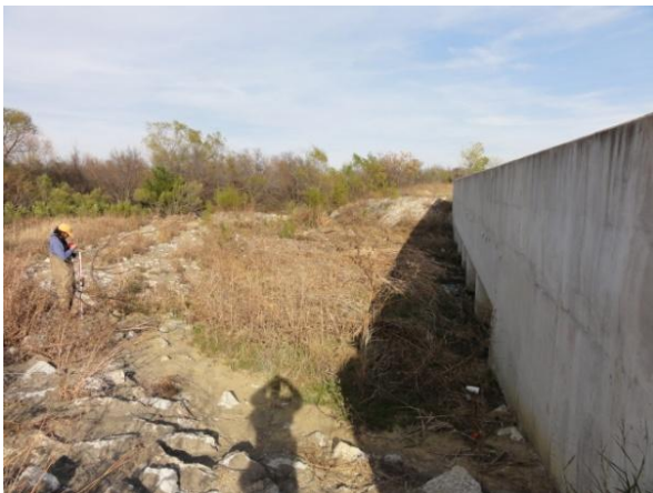
Polo Rd Crossing: Downstream Face
