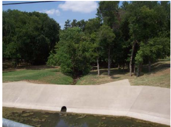
Carrier Pkwy Crossing: Looking Upstream
