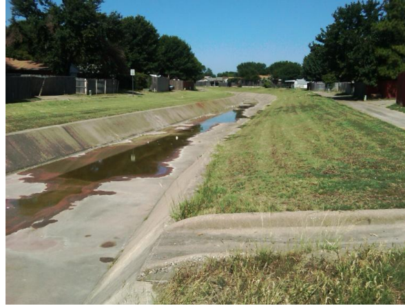
Matthew Rd Crossing: Looking Upstream
