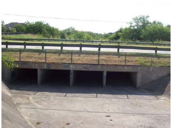
Robinson Rd Crossing: Upstream Face
