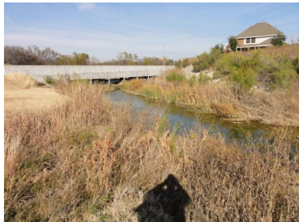
Polo Rd Crossing: Upstream Face
