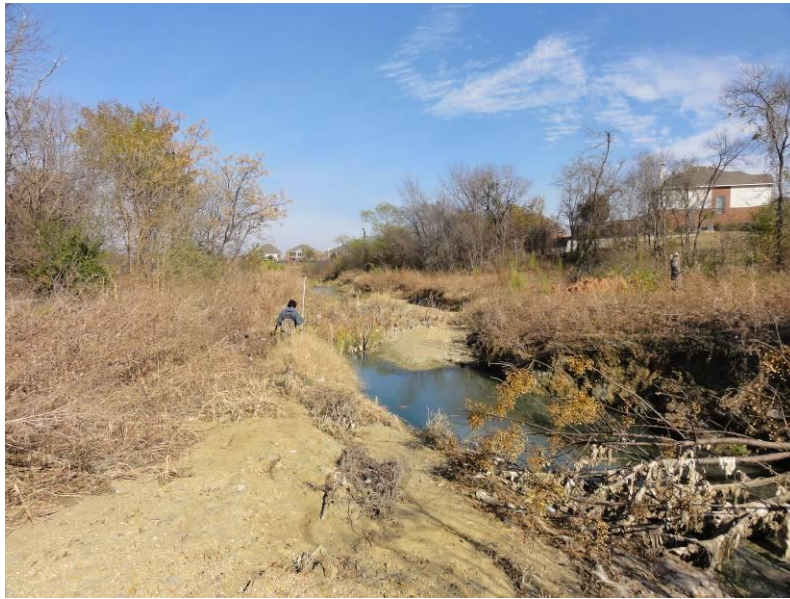
Figure 48. Zone of deposition and widening of the channel upstream of the drop structure.
