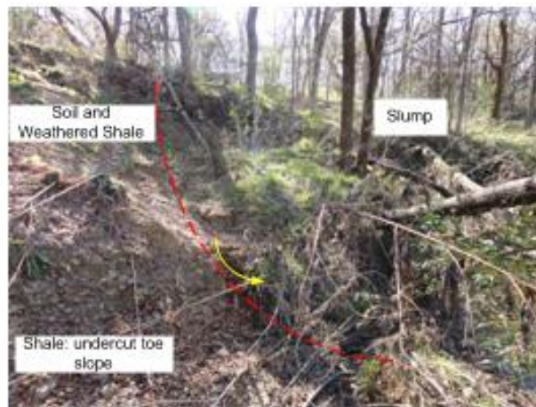
Figure 67. Slump type failure along Cedar Creek (Between Stations 11921 and 12 291). These failures are found where the slopes are typically less than 60 degrees and the stream cuts into an area where the shale is highly weathered or there is soil forming the channel banks. In this case, the slump appears to occur in the upper bank soil material above the shale bedrock. In most cases the failures will “bottom out” on top of the shale at the base of the weathered material.
