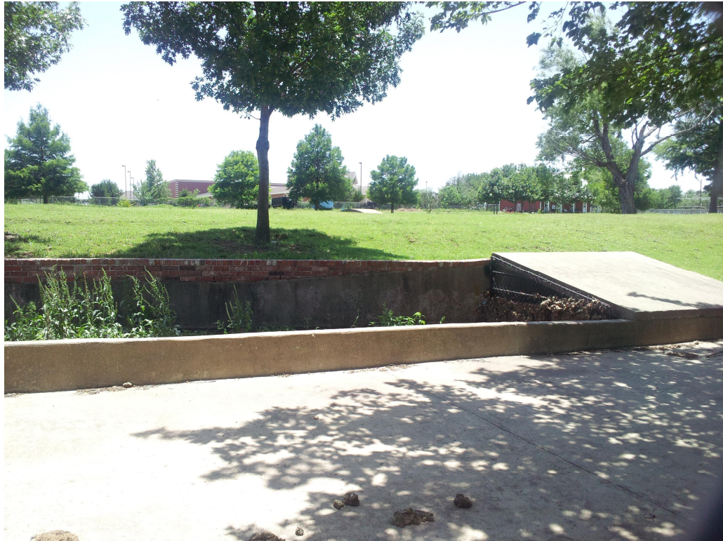
Figure X-4 – Detention Pond Outfall (facing South)
