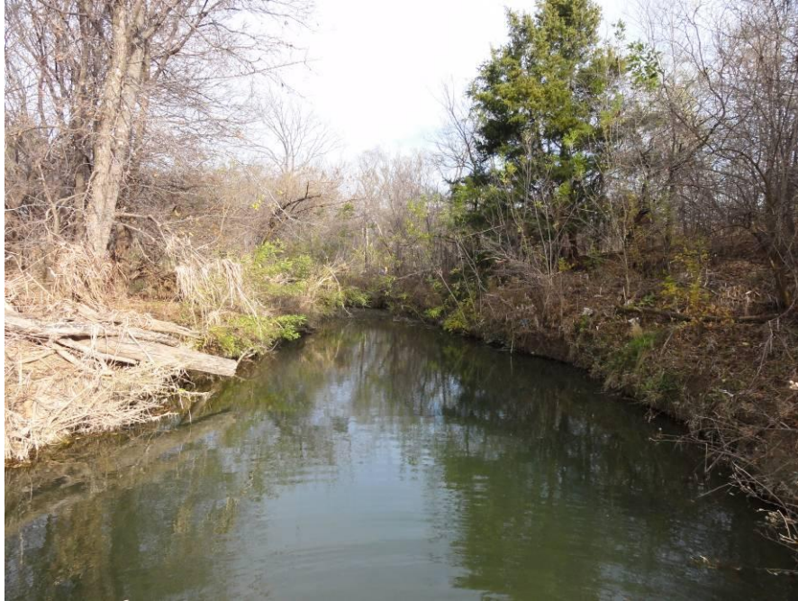
Figure 54. Pooled section immediately below the rip rapped channel downstream of Polo Rd.
