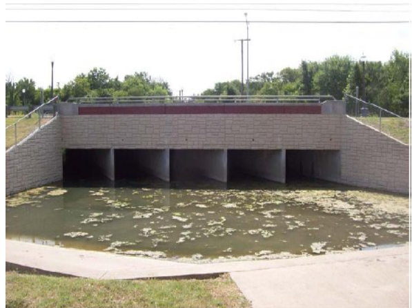
Carrier Pkwy Crossing: Upstream Face
