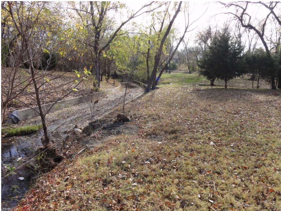
Looking downstream at concrete flume.
