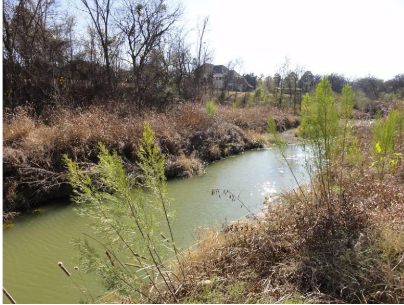
Figure 49. Stable banks and widened grassed channel above the drop structure.
