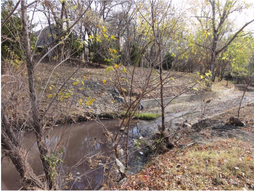
Looking downstream at concrete flume.
