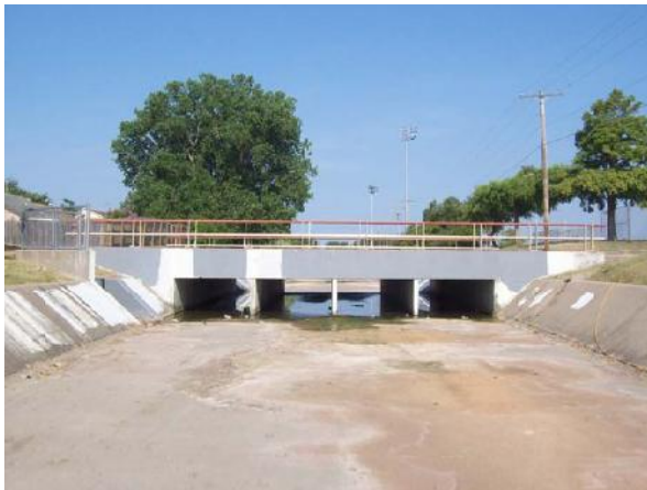
Prairie Rd Crossing: Downstream Face
