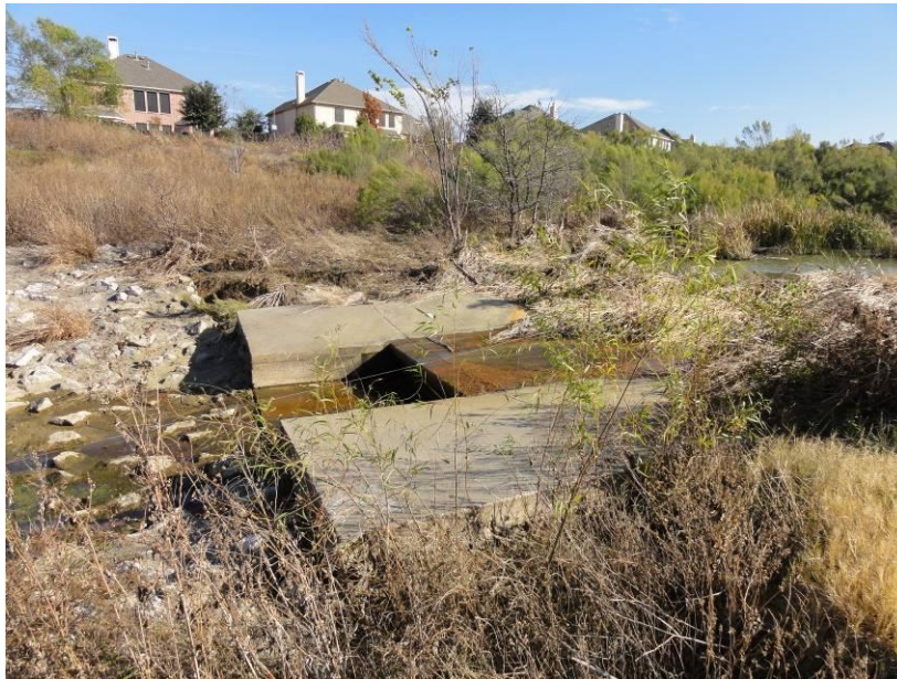
Figure 52. Lower hardpoint on the channel which controls the upstream grade.
