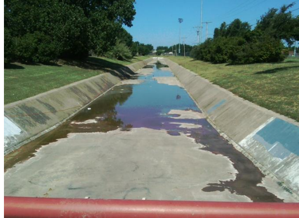
Prairie Rd Crossing: Looking Upstream
