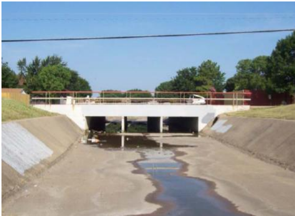
Matthew Rd Crossing: Downstream Face
