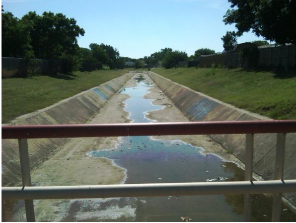
Matthew Rd Crossing: Looking Downstream
