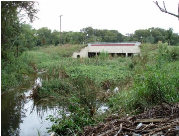
Carrier Pkwy Crossing: Downstream Face
