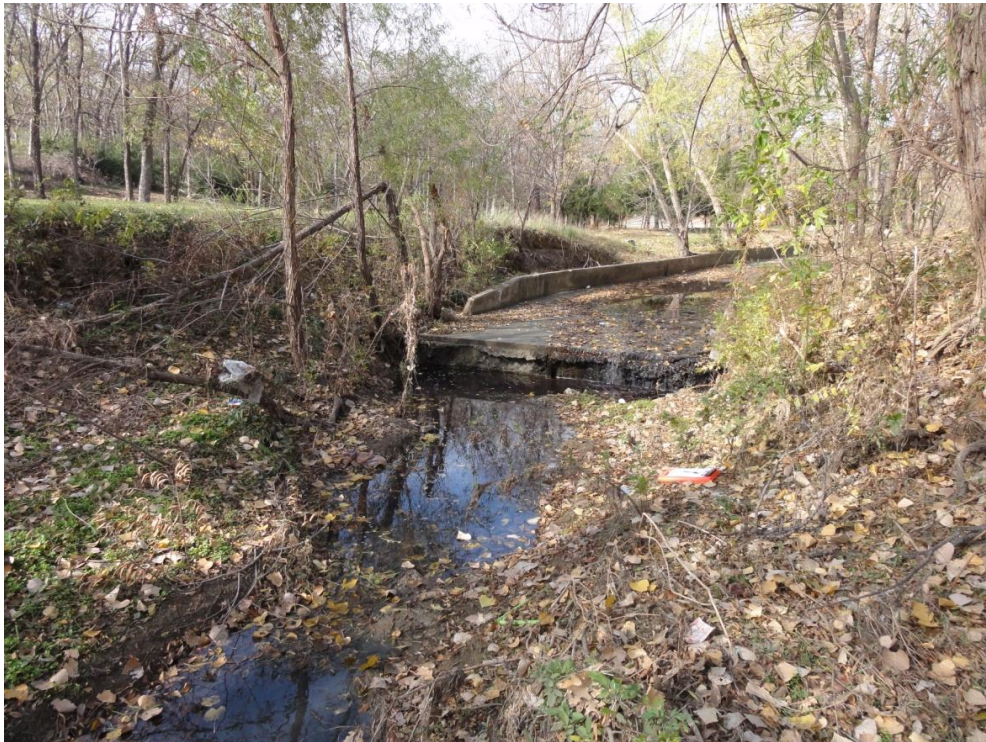
Looking upstream at the end of the concrete flume.
