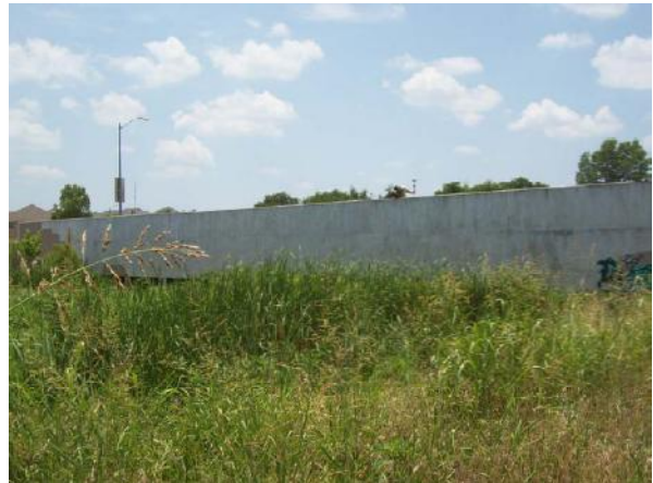
Bardin Rd Crossing: Upstream Face
