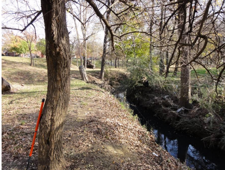
Figure 31. Incising channel downstream of concrete lined channel.
