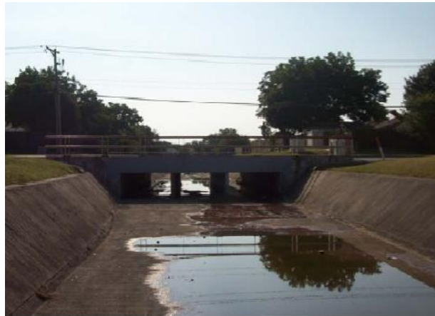
Matthew Rd Crossing: Upstream Face
