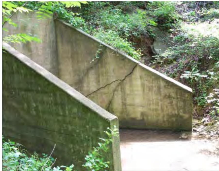
Picture XI-1 – Example of Structural Criteria (Photo ID 1613)
