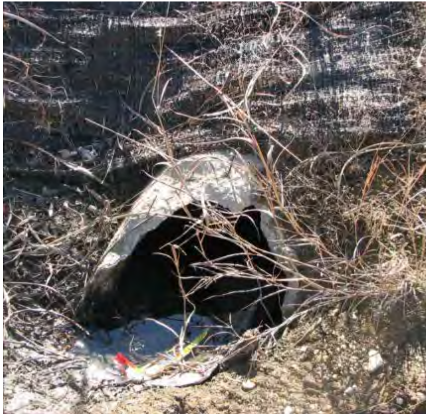
Picture XI-4 – Example of No Headwall Criteria (Photo ID 1613)
