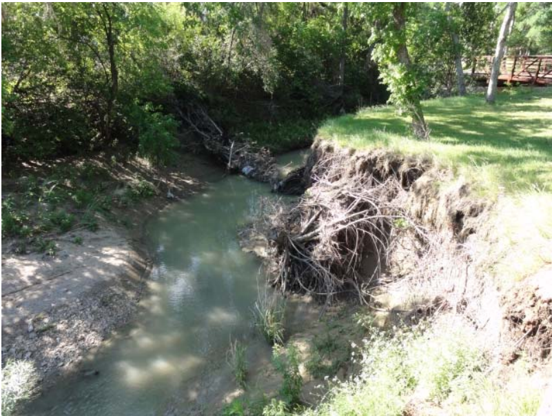
Figure IX-30. Typical Section of Degraded Channel in Waggoner Park (Station 6+25)
