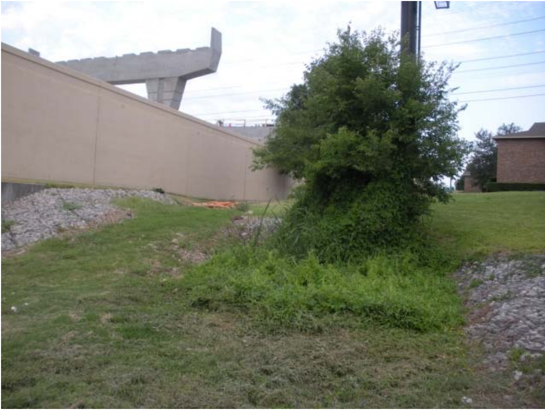
Photo of Combined Storm Drain Outfalls 26 and 27
