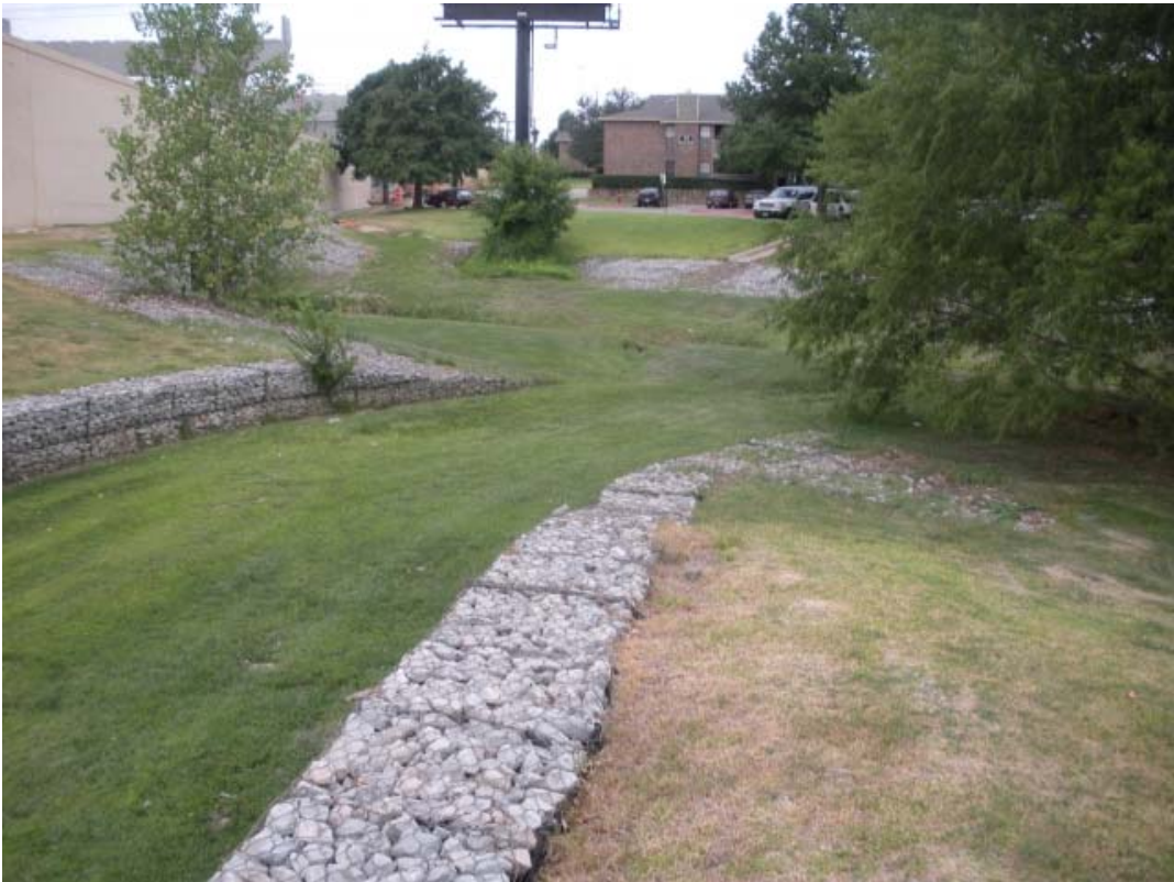
Photo of Storm Drain Outfall 28c
