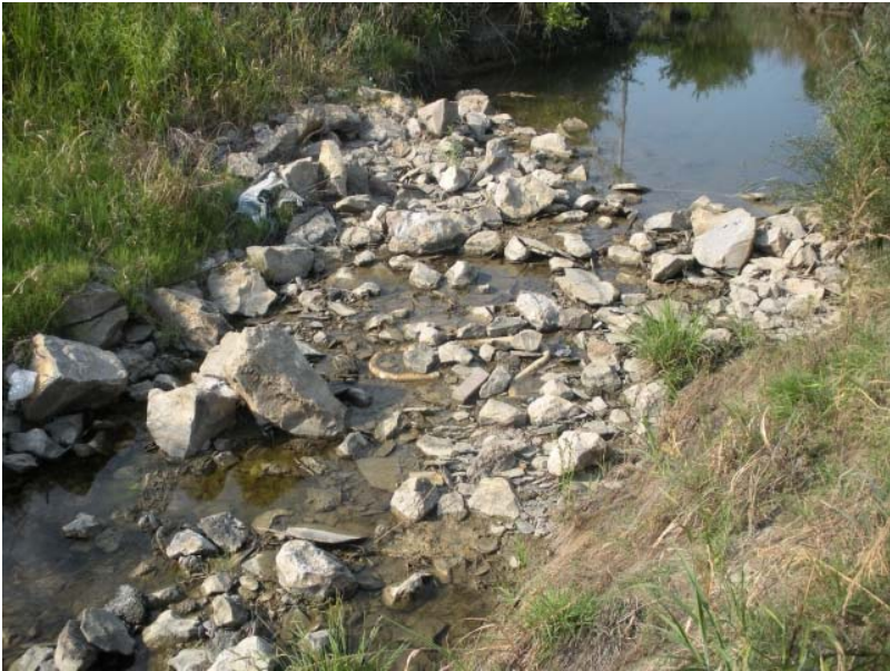
Figure IX-20. Loose Rock Riprap Drop Structure (Station 67+90)
