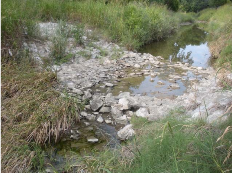
Figure IX-19. Grouted Rock Riprap Drop Structure (Station 78+00)
