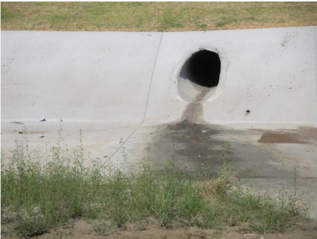
Photo of Storm Drain Outfall 14
