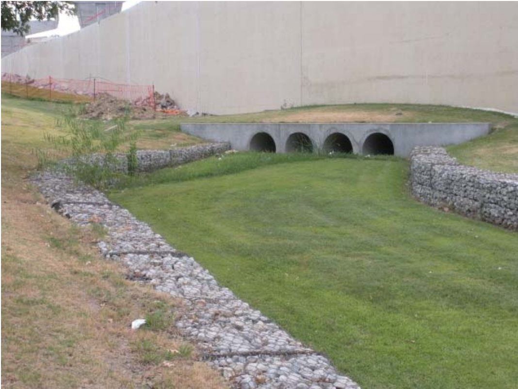
Photo of Storm Drain Outfall 28b
