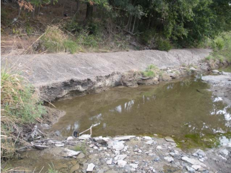
Figure IX-18. Exposed Sanitary Sewer Line Encasement (Station 82+30)
