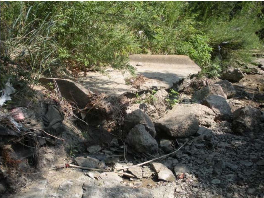
Photo of Storm Drain Outfalls 11 and 12
