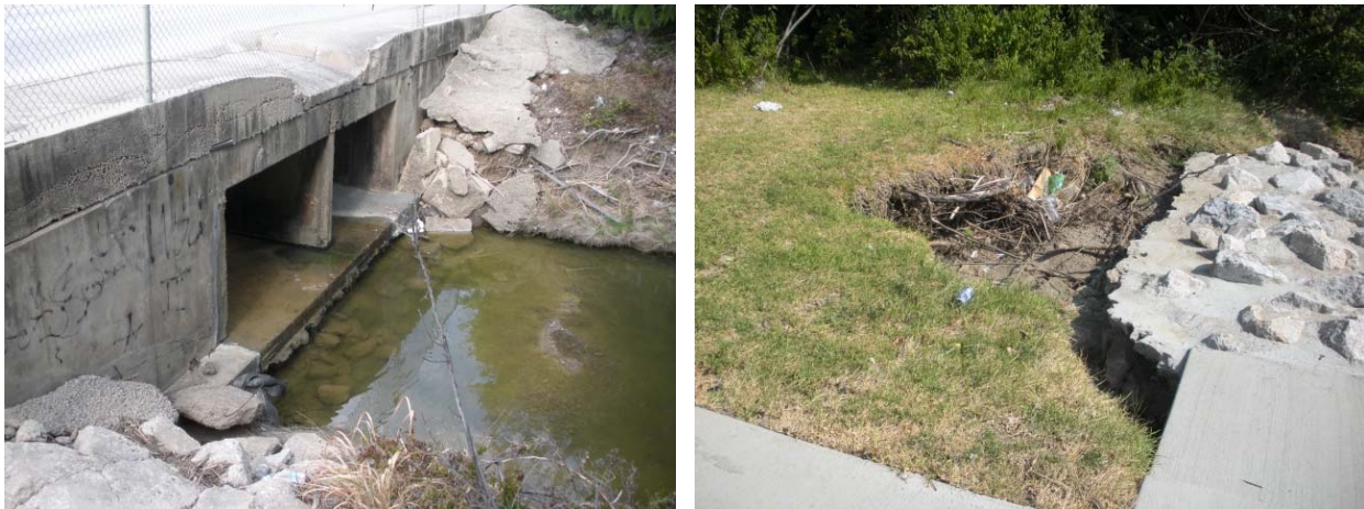
Figure IX-6. Typical Local Scour Problems at Tarrant Road (left), and Drop Structure Near Station 45+20 (right)
