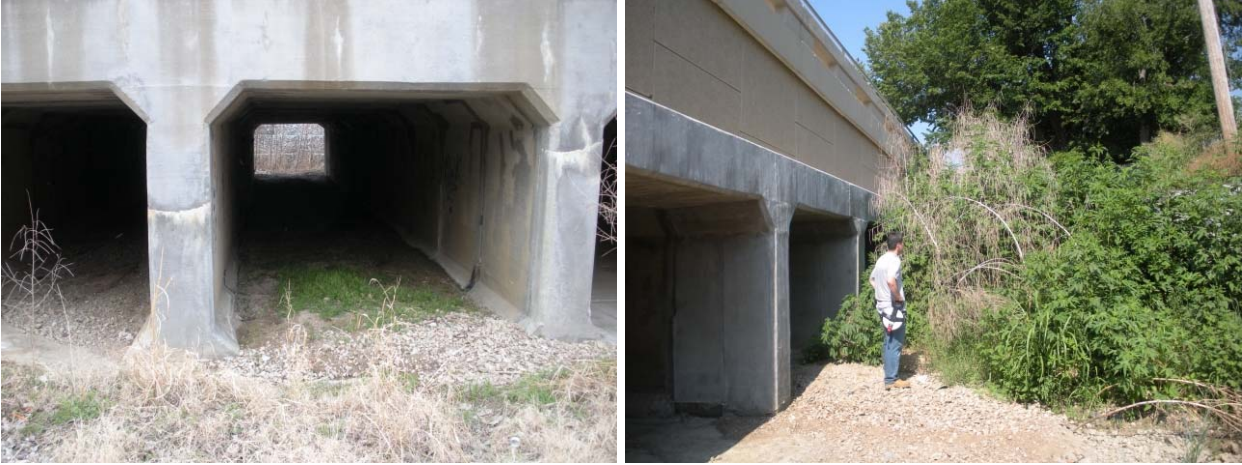
Figure IX-9. View of Sediment and Vegetation at the Egyptian Way Culverts.
