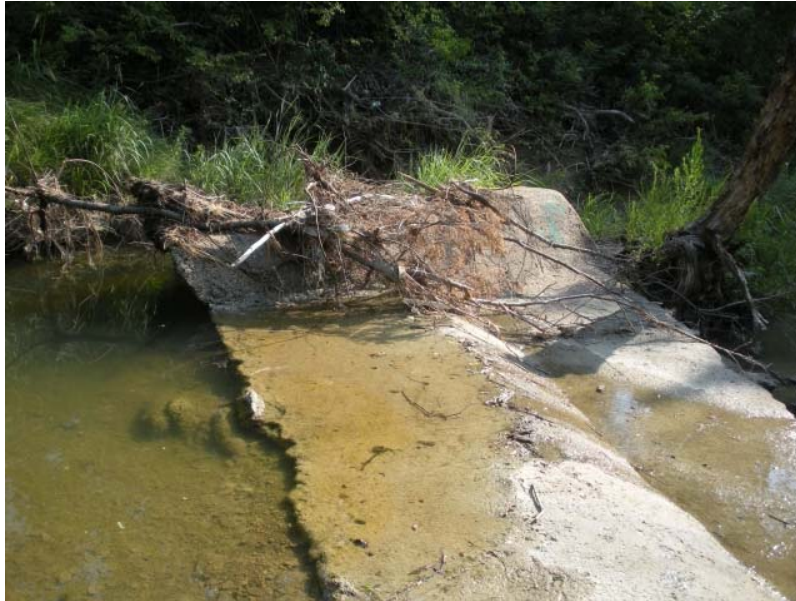
Figure IX-21. Encased Sanitary Sewer Crossing (Station 64+90)
