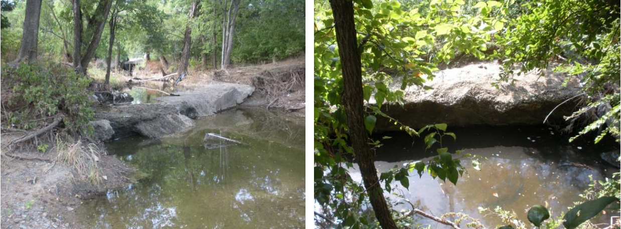
Figure IX-4. Views of Exposed Utility Encasements at Station 71+64 (left), and Station 35+50 (right).
