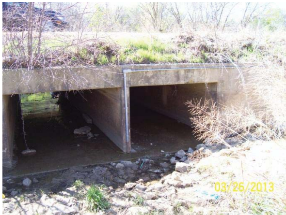
Camp Wisdom West Crossing: Downstream Face
