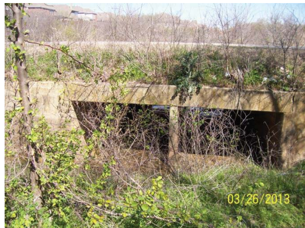
Camp Wisdom West Crossing: Upstream Face
