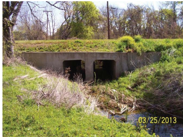
Robinson Rd Crossing: Upstream Face
