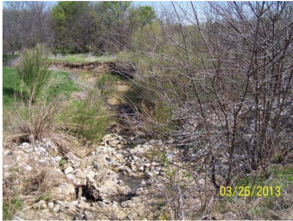
Camp Wisdom West Crossing: Looking DS
