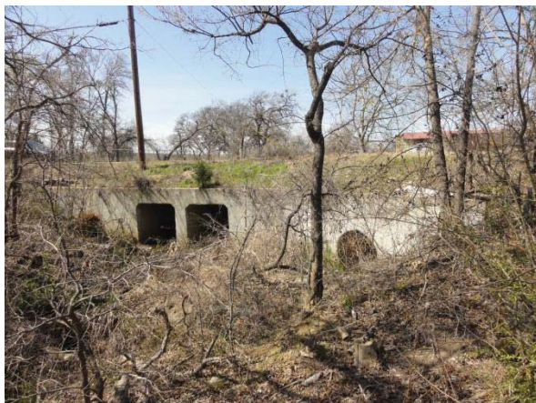
Robinson Rd Crossing: Downstream Face
