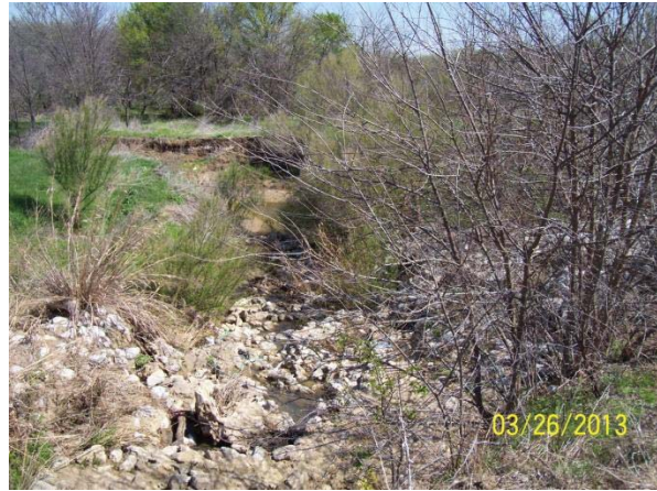
Camp Wisdom West Crossing: Looking US
